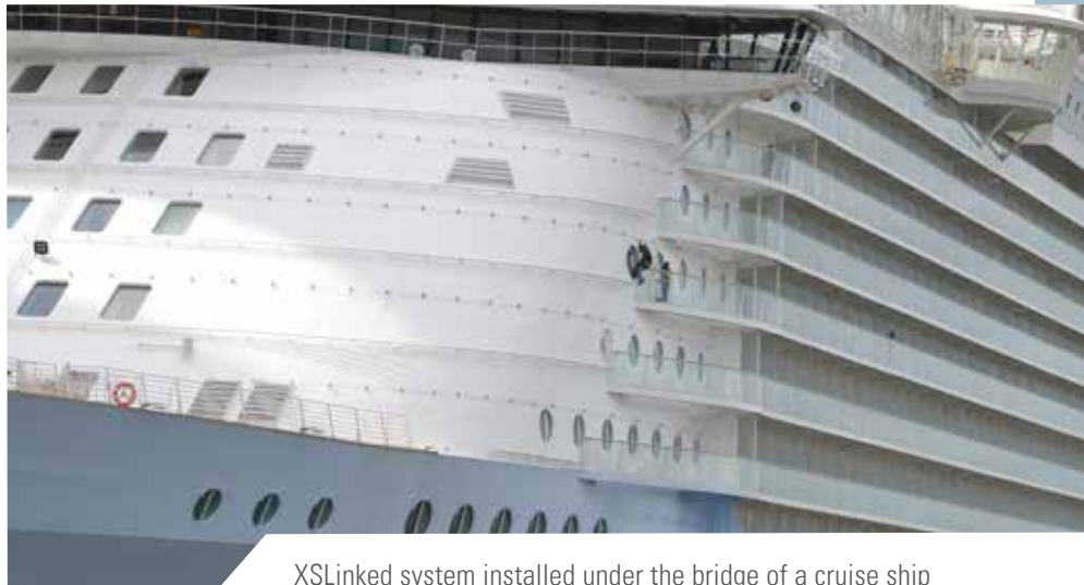
XSLinked system installed under the bridge of a cruise ship
